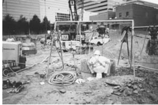
FIGURE 11-8 Setup for a shaft field inspection.
