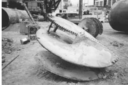
FIGURE 11-5 Large auger used in drilled shaft construction.
