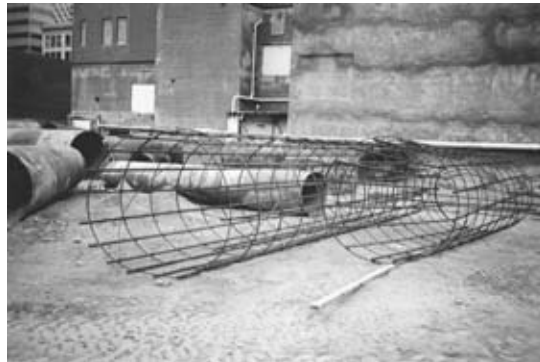
FIGURE 11-7 Reinforcing steel used in drilled shaft construction.
