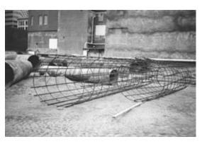
is poured. Normally, only the concrete in the upper part of the shaft is vibrated. It is always best to pour concrete in the dry, but if water is present, concrete can be placed underwater. Installation of reinforcing steel (see Figure 11–7) (if specified) should be carefully checked prior to placing concrete.
