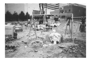
and concrete, and so on. Normally, the owner's representative should be present during construction of the shaft to ensure that it is done properly and according to specifications. Figure 11–8 shows a setup for a shaft field inspection.
