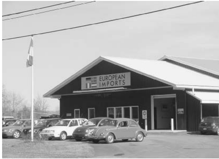
FIGURE 1-3 A product-specific service facility.
