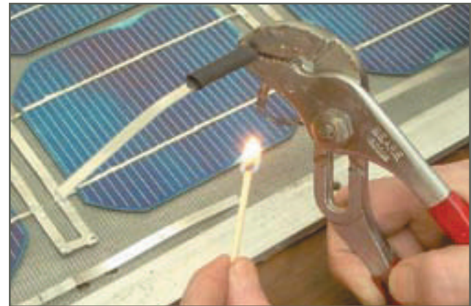
Use heat shrink tubing to insulate the leads.
