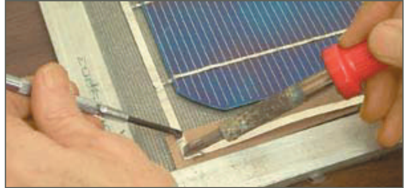
Solder the connection to the power take of leads.
