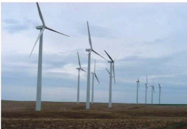
Wind turbines installed by IBEW Local 48 rise for miles in North Central Oregon.
