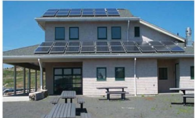
Solar panels installed by IBEW Local 103 atop the visitor's center on Spectacle Island in Boston Harbor.
