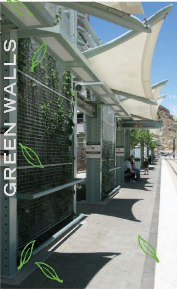
On twenty eight platforms greenscreen® green walls reduce radiating heat and help provide a cooling microclimate on the Metro Light Rail, Phoenix, AZ.
