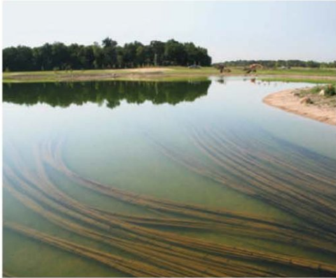
Sherman Health's runoff-retention pond doubles as a 15-acre water-source loop. The 650,000-square-foot facility expects to save $1 million a year in heating and cooling costs.
