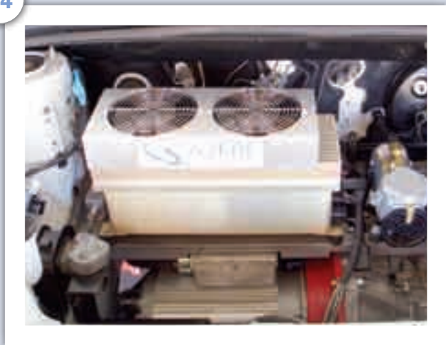
14. The Azure digital motor controller (DMOC) mounted. 15. The AC battery charger mounted in the trunk. 16. Programming the DMOC via a laptop.
