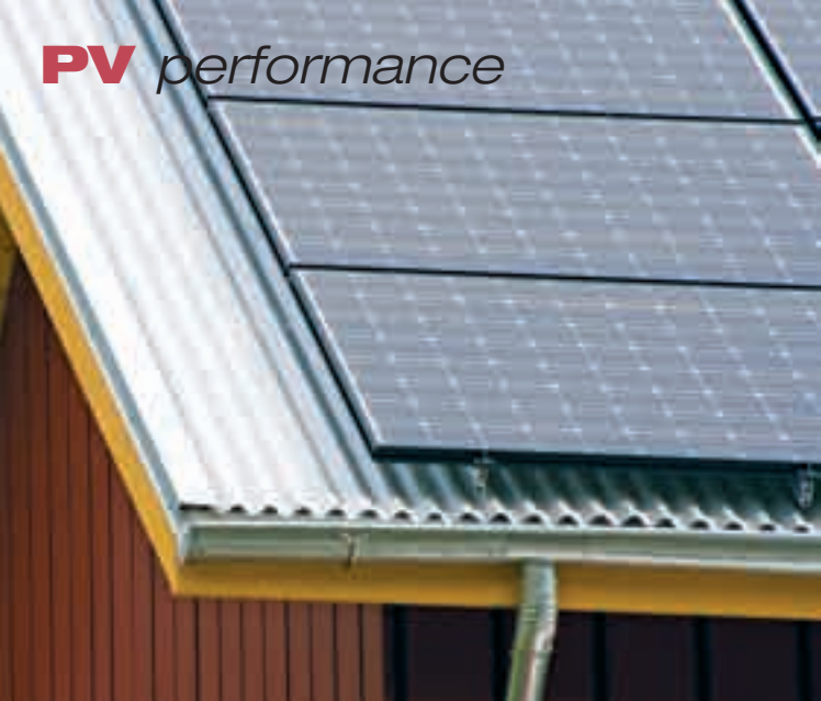
Roof standoff height—the space between the back of the module and the roof—affects air circulation, and thus cell temperature and performance.
