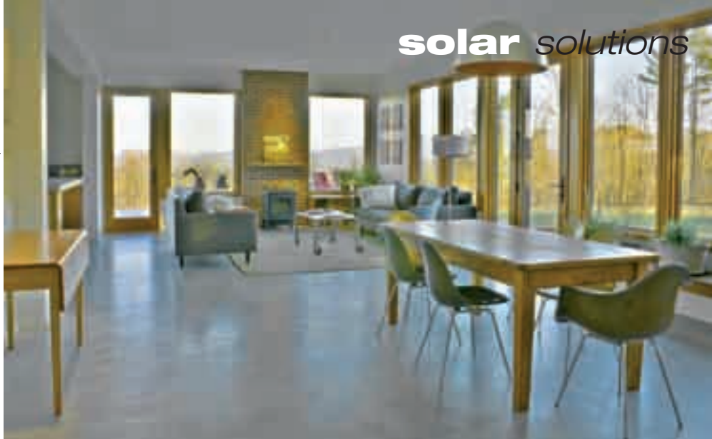
Large, south-facing windows admit solar gain, while the thermal mass in the concrete floors absorbs, stores, and reradiates the solar resource for wintertime heating.
