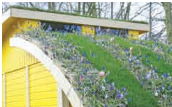
Living roofs are especially attractive for the home heating and cooling savings they can offer.
