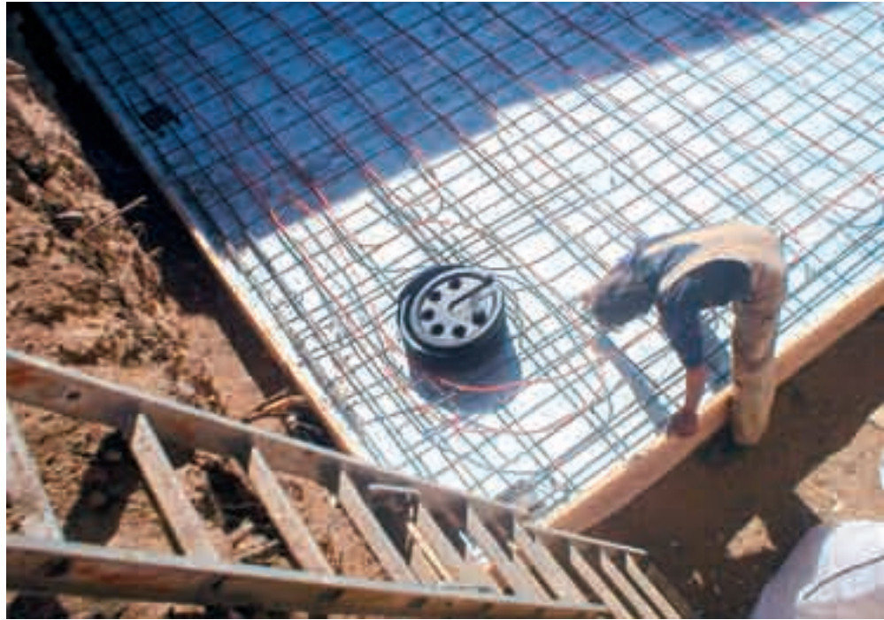
Insulating the entire slab with rigid foam is a better approach than insulating only the perimeter when using radiant-floor heating.
