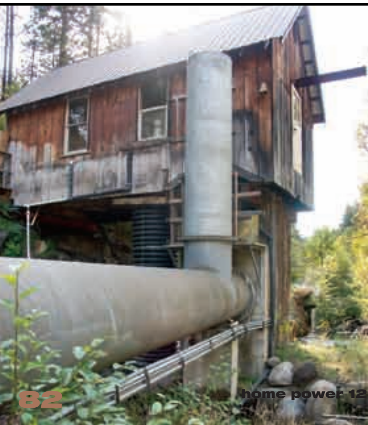
The penstock terminates at the powerhouse.
