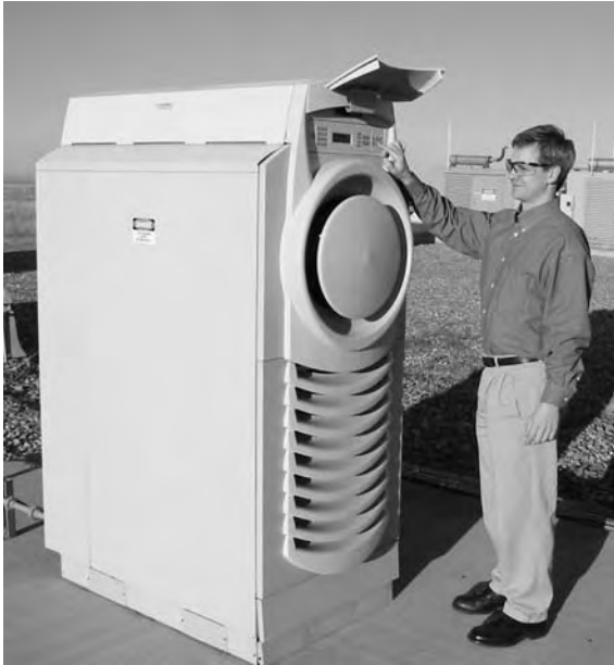
Figure 9.3 Capstone single-shaft microturbine. (Courtesy of National Renewable Energy Laboratory.)
