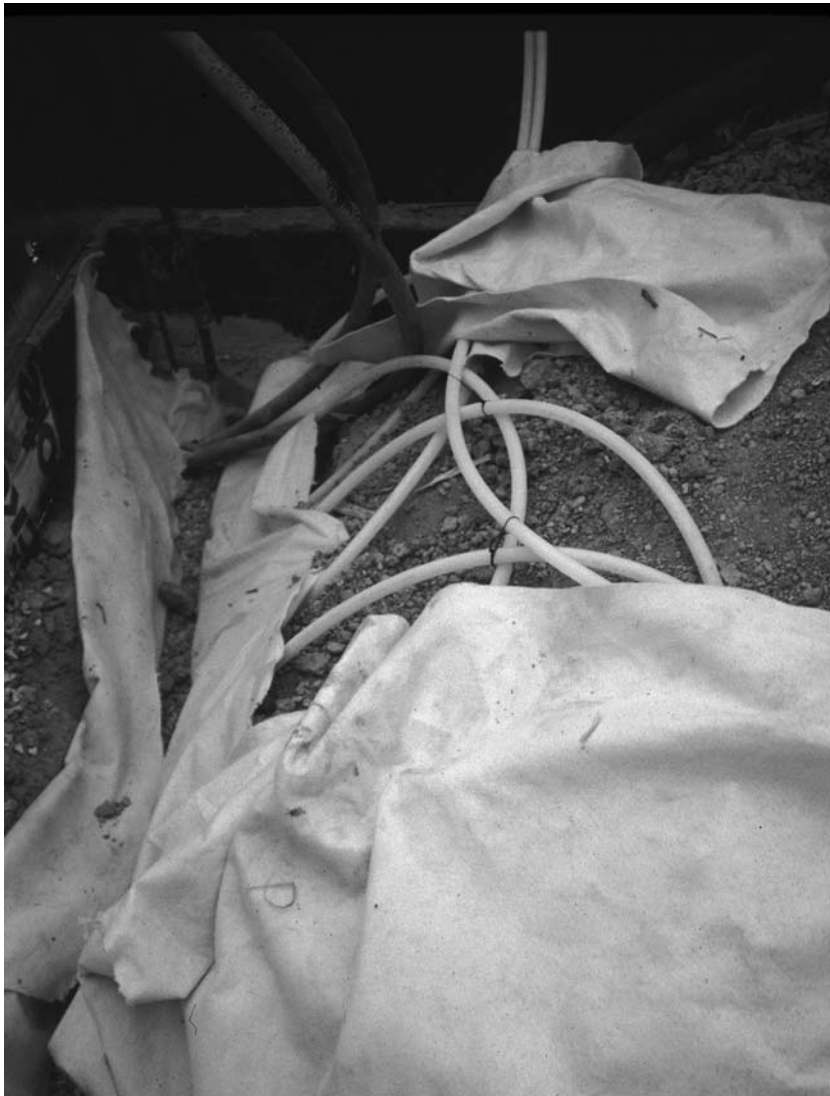
Figure 7.7 Photograph showing installation of ground coils.
