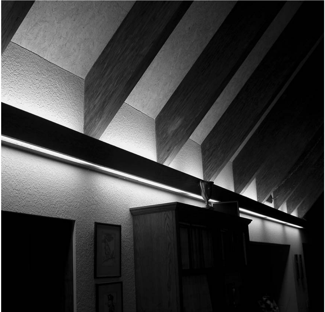
Figure 7.13 Photograph showing soffit lighting of ceiling rafters.
