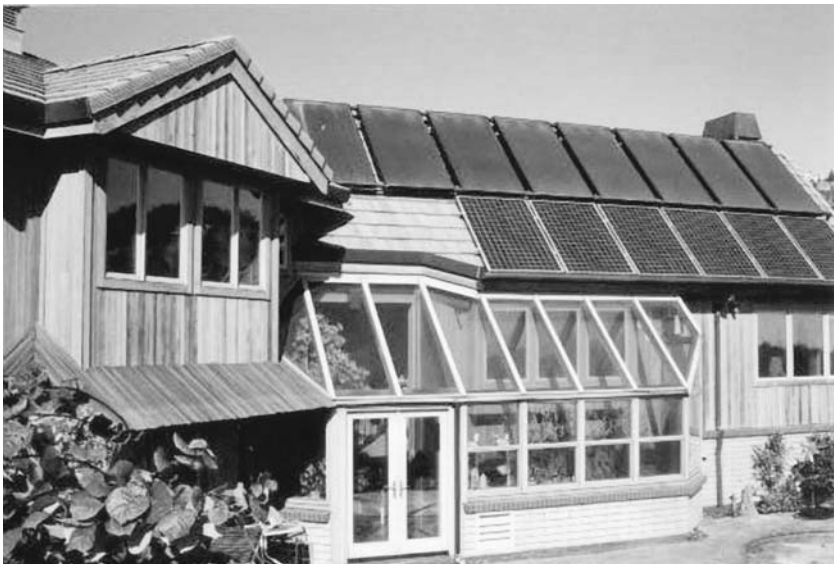
Figure 1.5 Completed Berkeley Solar house configuration.
