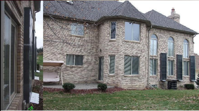
Reflector panel is optional, it adds about 5% more heat. Here it is shown with AOL garbage discs instead of an acrylic mirror.
