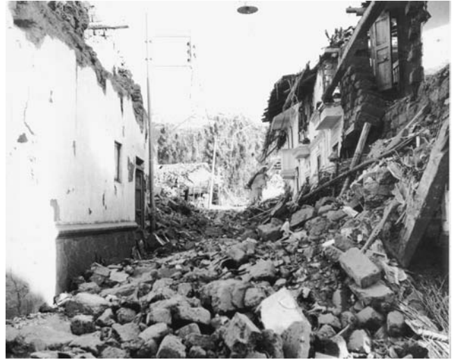
Massive destruction of adobe houses in the town of Hurez during the 1970 earthquake, by far Peru's worst natural disaster (Courtesy of the USGS)
