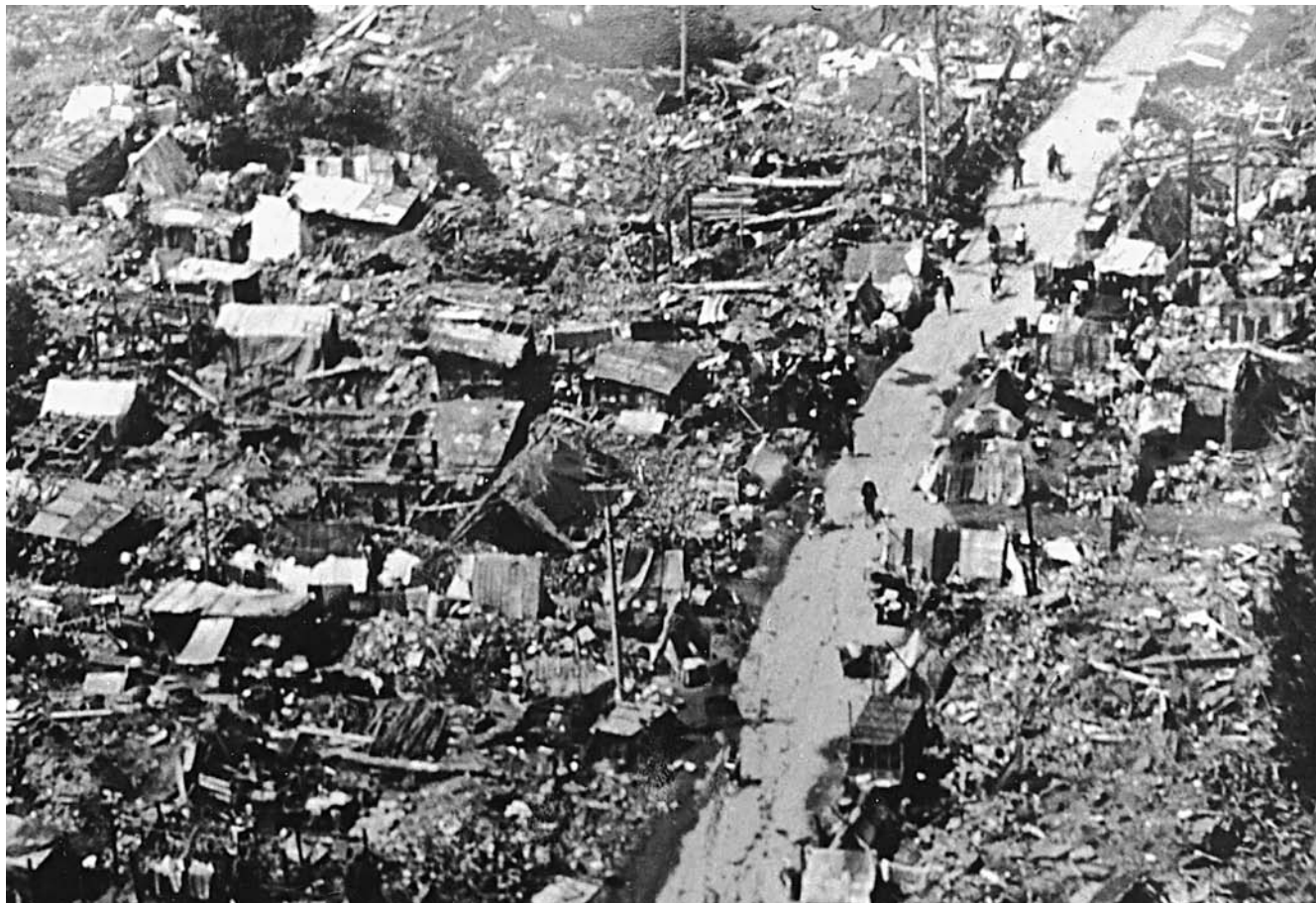
Complete destruction of all buildings (only tents for refugees are visible) by the great 1976 Tangshan earthquake. (Courtesy of the USGS)
