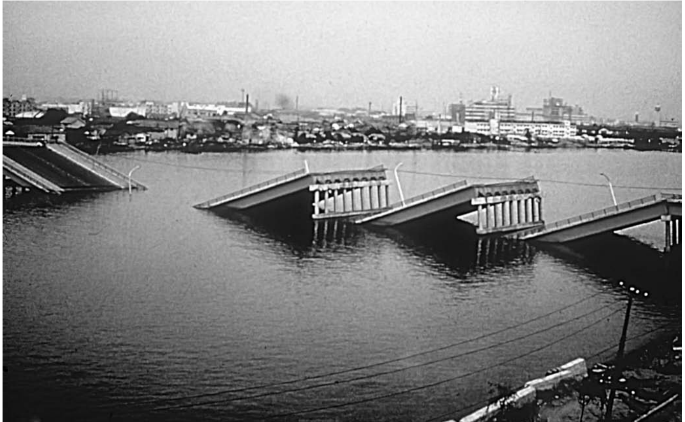
A collapsed bridge after the June 16, 1964, earthquake in Niigata, Japan. The earthquake of magnitude 7.4 killed 26, injured 447, and damaged 9,750 structures in Niigata. Two piers on this bridge collapsed, and successive spans were pulled away from piers as the bridge was pulled apart. (Courtesy of NOAA)
