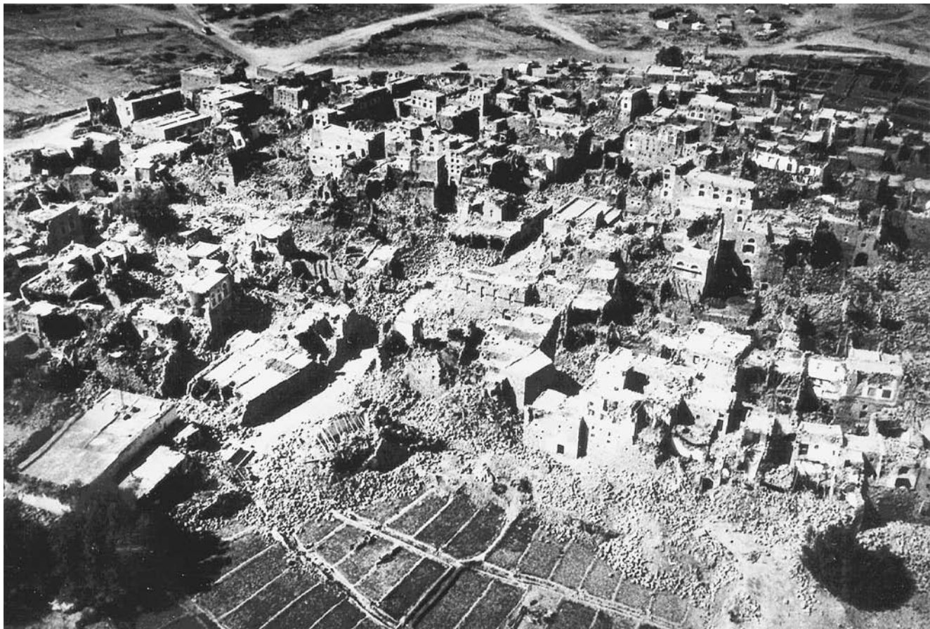
Damage to buildings as a result of the Dhamar, Yemen, earthquake in 1982 (Courtesy of the USGS)
