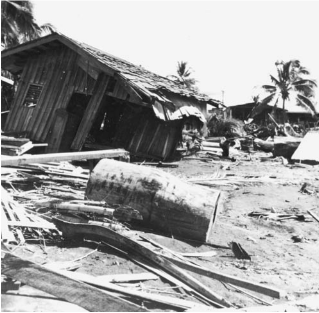
The resulting tsunami from the 1976 Moro Gulf earthquake produced extensive damage such as this at Lebak, Mindanao. (Courtesy of the USGS)
