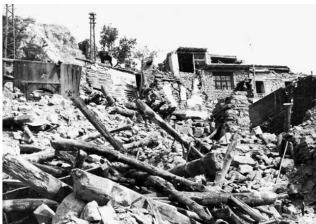
The total collapse of a house in Lice, Turkey, as a result of an earthquake in 1975 (Courtesy of the USGS)
