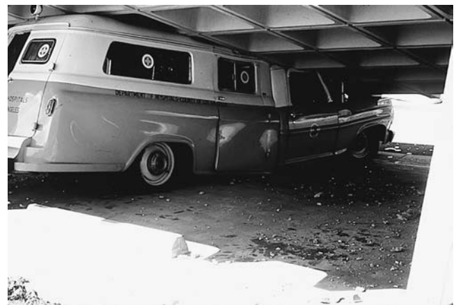
This and other ambulances, crushed by the collapse of the Olive View Hospital, Los Angeles, were rendered useless for rescue operations after the 1971 San Fernando earthquake in southern California. (Courtesy of the USGS)
