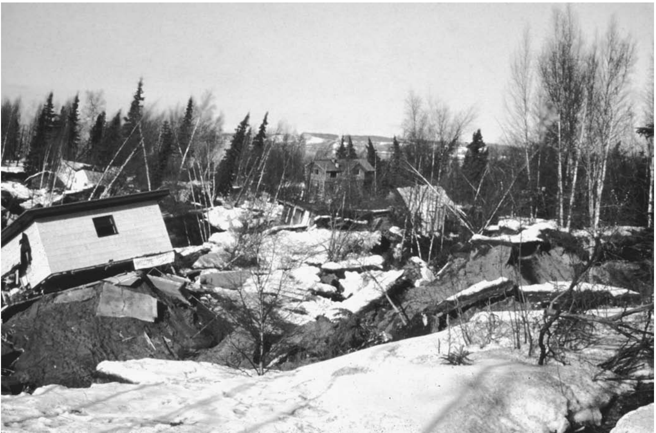
Chaotic jumble of houses, trees, and landscape resulting from slumping and surface failure during the 1964 Good Friday earthquake in Alaska (Courtesy of the USGS)
