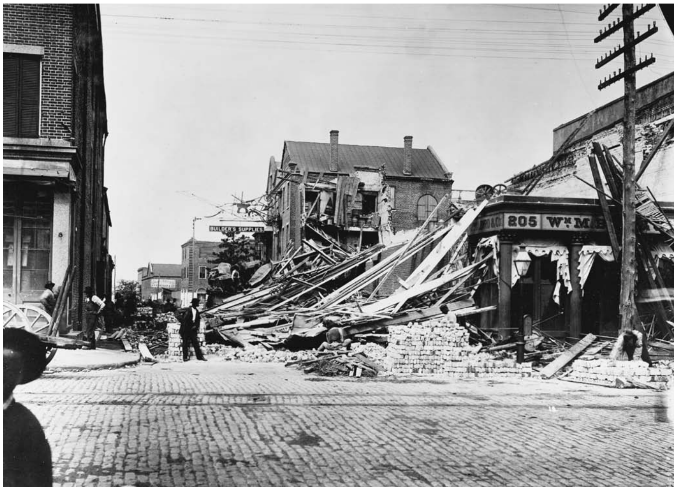
Collapsed buildings litter the street in Charleston, South Carolina, after the 1886 earthquake. It was the strongest historical earthquake on the east coast of the United States. (Courtesy of the USGS)
