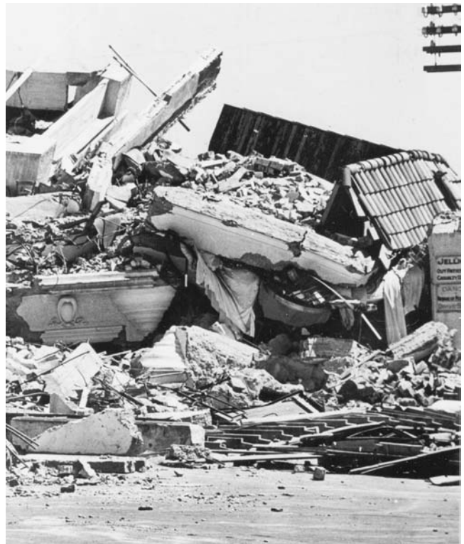
The nurses' home at Napier Hospital was a pile of rubble after the 1931 Napier (Hawke's Bay) earthquake. (Courtesy of the USGS)
