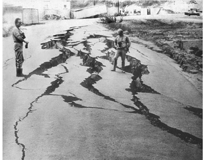
Fissures in a paved road at the head of a slump block generated by the 1970 Nevados Huascarán earthquake in Peru (Courtesy of the USGS)
