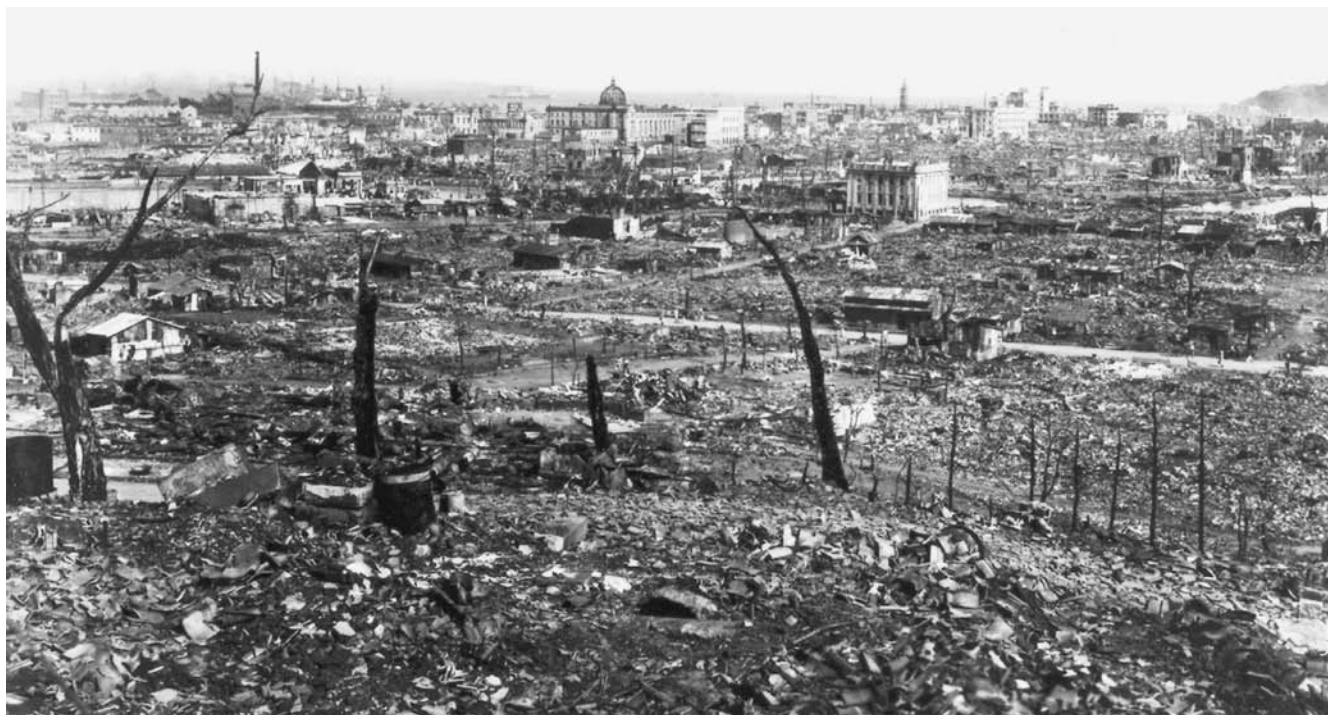
Only the sturdier buildings of downtown Tokyo, Japan, such as the Imperial Hotel (closest building, to right), survived the massive 1923 Kanto earthquake and resulting fires. (Courtesy of the USGS)
