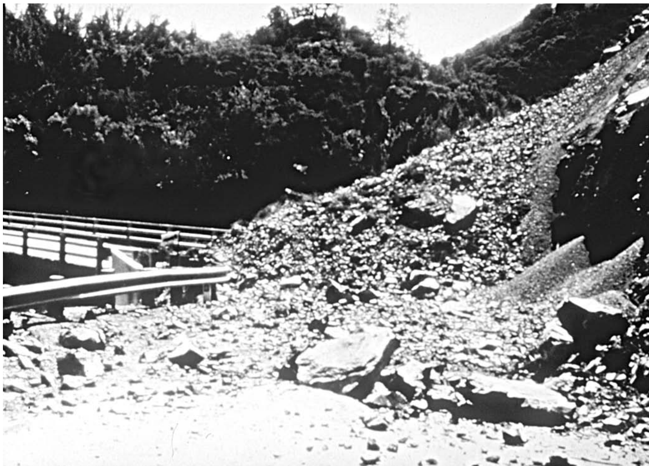
Rockslide blocks destroy a highway after the April 24, 1984, earthquake in Morgan Hill, California. The earthquake had a Richter magnitude of 6.2 and caused $30 million in property damage. (Courtesy of NOAA)
