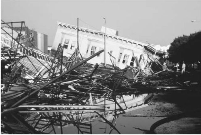
The Marina district of San Francisco, California, suffered much worse destruction than the rest of the city during the 1989 Loma Prieta earthquake. The destruction shown here at Beach and Divisadero Streets is a good example. (Courtesy of the USGS)
