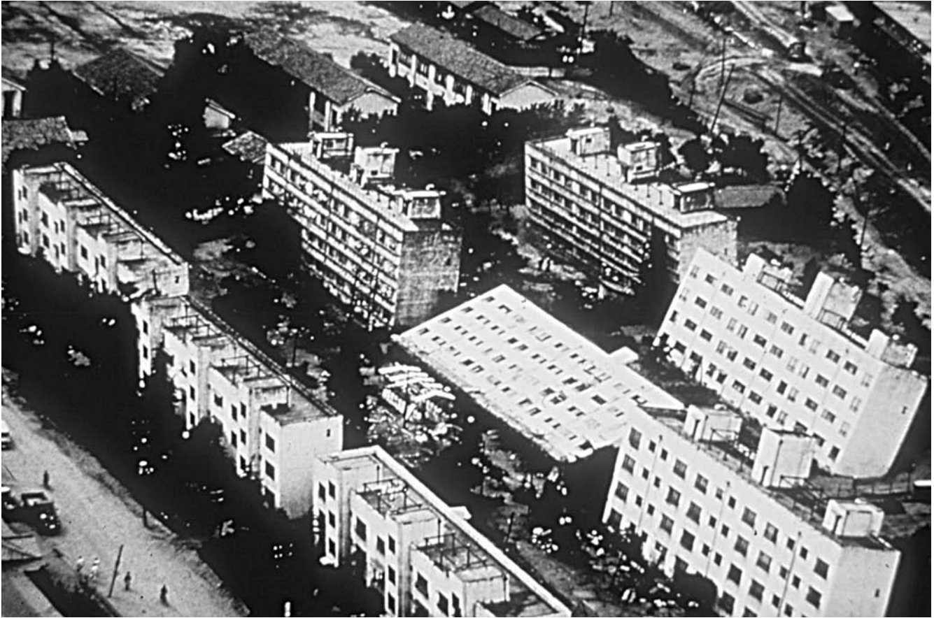
These apartment buildings in Niigata, Japan, were built to be earthquake-proof. During the June 16, 1964, earthquake of magnitude 7.4, the buildings withstood the shaking, but liquefaction compromised the foundations, and the buildings fell over still perfectly intact. (Courtesy of NOAA)
