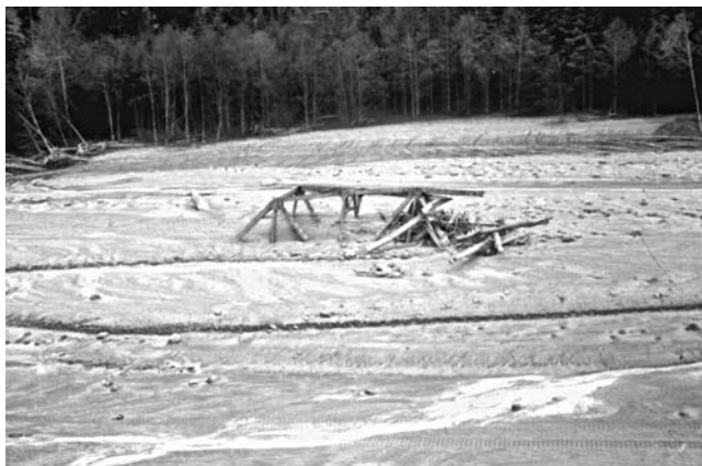
Mudflow/lahar from the Mount Saint Helens eruption, May 18, 1980. The mudflow came down a river valley and destroyed a bridge. It filled the old river with mud. (Courtesy of the USGS)
