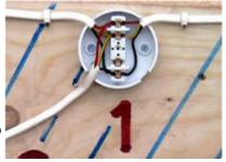
Top cables are existing, cut and joined. Bottom cable goes to second junction box. Your complete circuit should look like this...only a bit more spread out!
