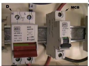
be a 20 amp MCB, 30 amp fuse = 32 amp MCB and a 45 amp fuse must now be a 40 amp MCB.
