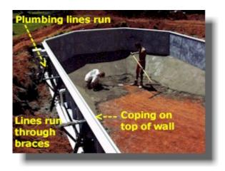
Start placing and finishing the 2" cement mixture at the deep end as shown. Start at the top of the diving well slopes, working your way toward the bottom drain. Use a wood or metal concrete finishing tool. The correct finish is smooth and flat....not beautiful.
