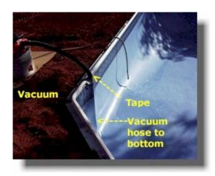
Open up a small section of the liner at the top and insert shop vacuum as shown. Vacuum hose should reach to bottom of pool. Duck tape closed the liner/hose opening. Turn on vacuum and it will pull the liner tighter to the sides of the pool. Smooth out any wrinkles. Vacuum should run until their is 8" of water in the shallow end.
