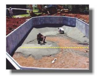
If you have in-the-wall steps, curve the cement bottom up on the plastic front piece of the step unit with a 2" radius. In other words add extra cement where the step unit meets the bottom, and smooth it up the front wall of the step unit 2". The vinyl liner has trouble stretching into this bottom corner of the pool, so it is being filled in.
