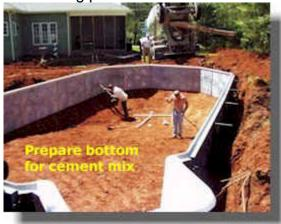
**Step9:** While preparing the bottom in step 8, also dig out for the bottom drain in the center of the deep end diving well as shown in various pictures. Make the drain box 2" above the excavation level of the soil.
