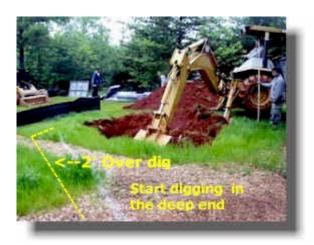
**Step 4:** The pool kit you purchase will provide the measurements for the final size of the pool bottom and sides. You will aim to **over dig** the sides of the pool approximately 24" bigger than your outline marked on the ground when you started. This provides working room for the panels, room for the panel braces shown in the picture to the right, and is where the concrete footer is poured that holds the bottom of the panel and panel braces.
