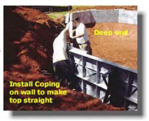
**Step 6:** After your satisfied the pool panels are level (you can shim up low spots with pieces of brick or block) then run string along the top of straight runs and adjust wall braces to make the top straight.
