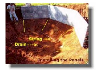
**Step 3:** On the big day...start digging in the deep end. The pattern of the dig follows the diagram below. (which is a top, side and end view of the pool)
