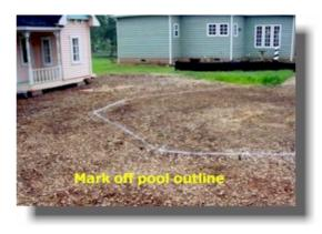
**Step 2:** Mark off the outline of the pool with stakes and string so that you can do fine tuning of final pool placement. Call for underground utilities to be marked (free service) so that you will not dig or trench through a buried cable or line. Secure your building permit. Determine supplier of pool and purchase pool kit, liner, Portland cement, vermiculite and all necessary supplies such as sliding board, pool vacuum etc. (These will be covered later)
