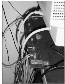
Figure 13-10: A copper ground bus installed in my shack.
