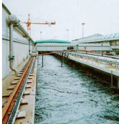
**Fig. 8.63.** By injecting  $\text{FeCl}_3$  into the sludge, dissolved phosphate precipitates from the waste water
