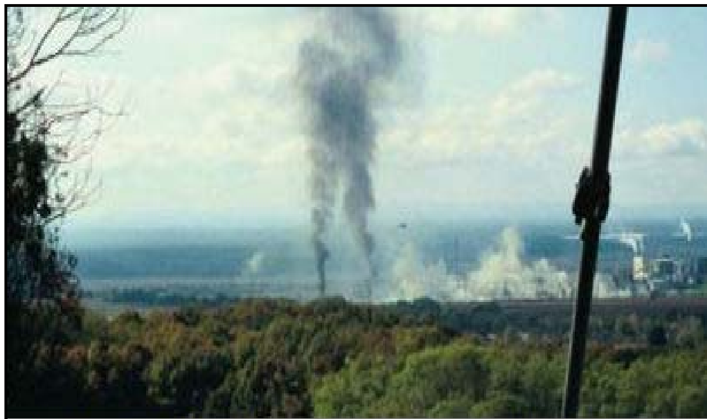
Figure F-7. Petrochemia chemical plant under attack by Serbian forces.
