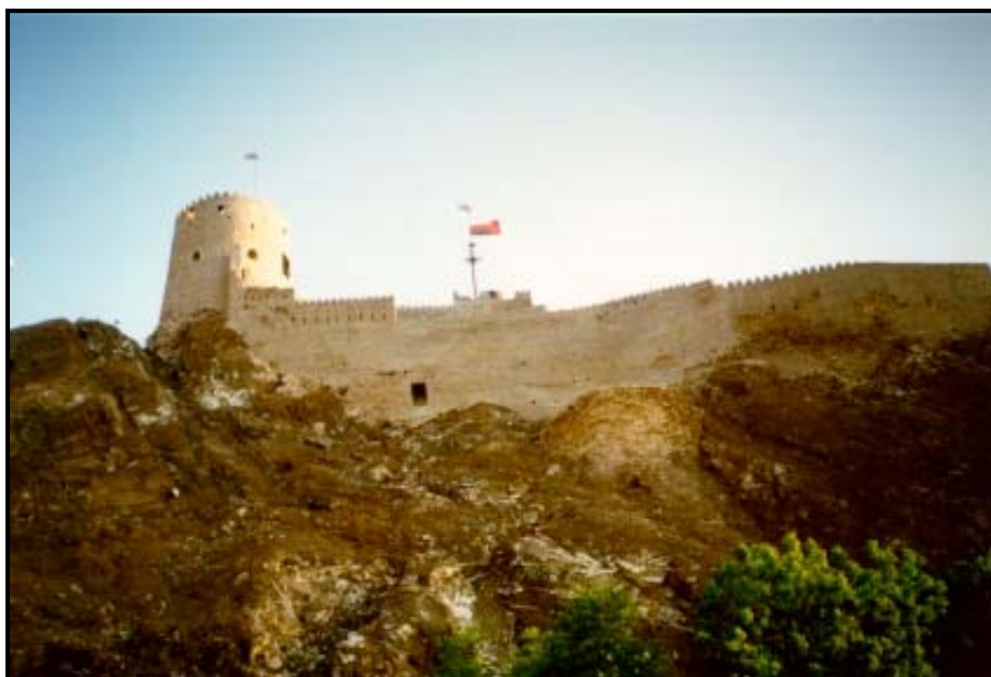
Figure 2-9. Permanent or fixed fortifications.
