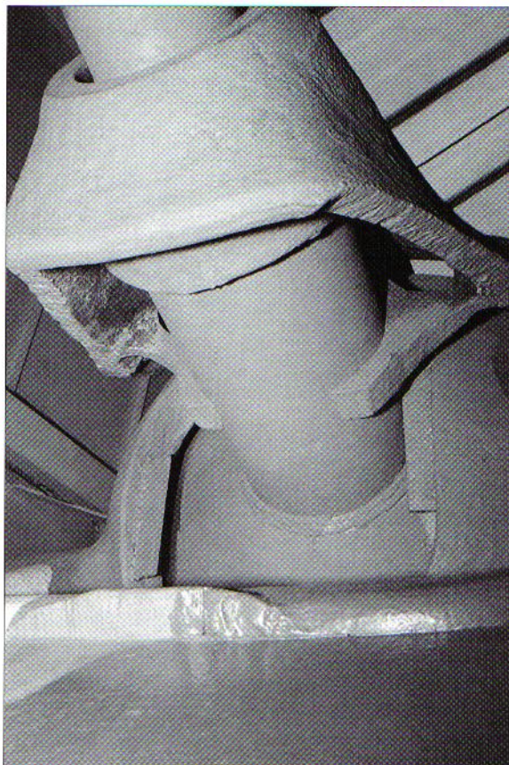
Close-up detail of the gun mantel of Fgst.Nr.322111. (HLD)
