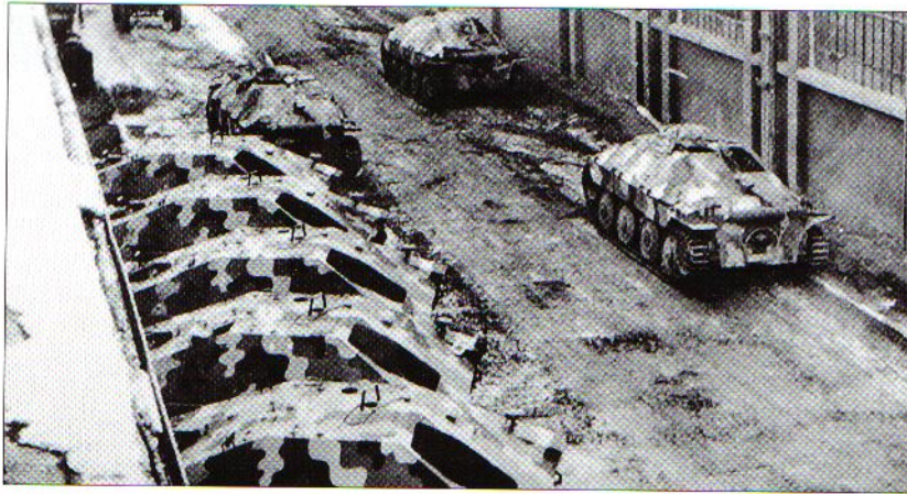
Pre-painted hulls and partly completed Jagdpanzer 38 at BMM in October 1944. The visible features of the Jagdpanzer 38 of this period were: the new driver vision block arrangements; wheels with 16 rivets; new hulls with the underside of the tow brackets notched and rear brackets lowered. The front and rear of the Schürzten was bent inwards to avoid catching and being torn off. In October the camouflage pattern at BMM was changed to a base of Dunkelgelb – RAL 7028 (dark yellow) with patches and stripes of Olivgrün – RAL 6003 (dark olive green) and Rotbraun – RAL 8017 (dark red brown). Matt black rectangles were painted on the front plate as decoys to protect the driver's vision blocks. (BMM)
