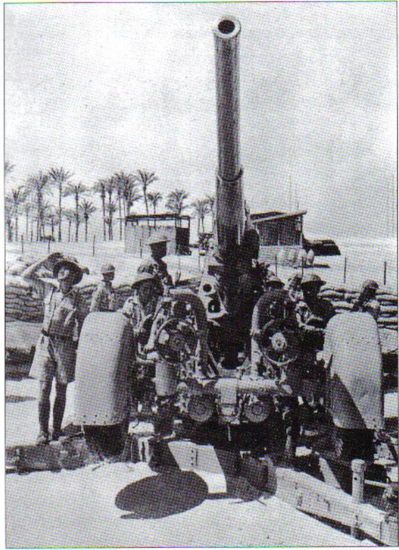
ABOVE The business end of a 3.7in HAA gun. The gun's axles were removable, but if retained they made rapid redeployment easier during the fluid engagements that typified the campaign in the desert. This piece is manned by gunners of the Malta Artillery, who were normally only required to serve within their home islands, although a small number of volunteers served overseas.
