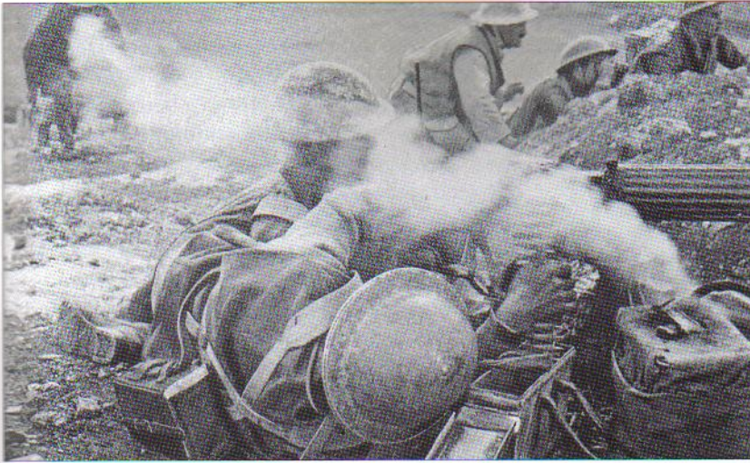
A Vickers MMG crew in action. A cloud of steam billows from the condenser can during sustained fire; despite this obvious fluid loss the condenser did save some of the precious water, which was then poured back into the gun's cooling jacket. Each of the three brigades of an infantry division usually had one company of the divisional MG battalion attached in support.
