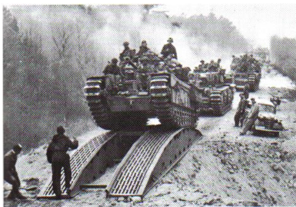
The 30-foot bridge carried by the Churchill bridgelayer was also used to reinforce cratered roads.
