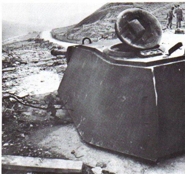
Carefully sited Panther turrets on concrete casemates were encountered in the Hitler and Gothic Lines.
