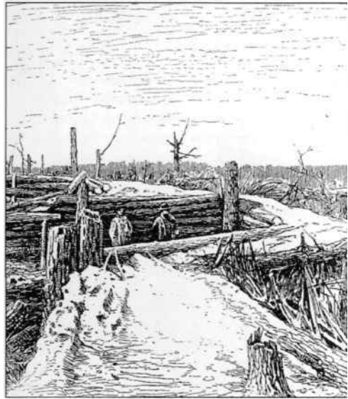
Confederates used felled trees covered with earth to fabricate an intricate set of field fortifications unlike anything that had been used earlier in the war. This view is in the vicinity of the nose of the Mule Shoe, near what became 'the Bloody Angle.' (Public domain)
