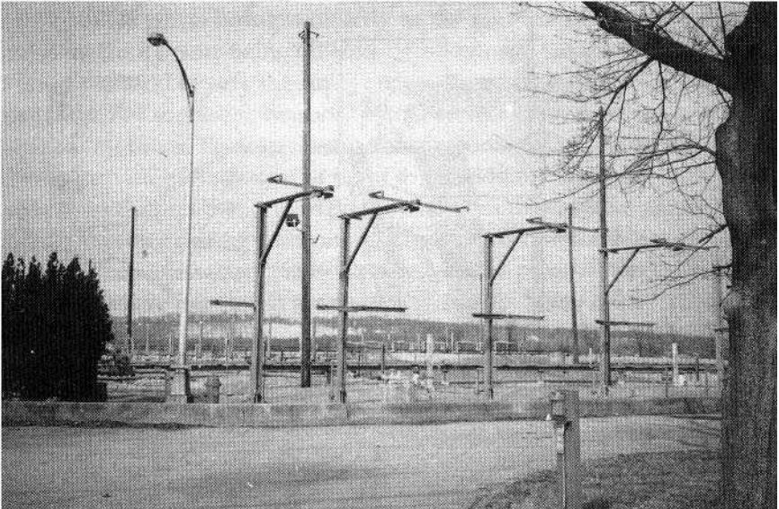
Figure 3-4. Buried Gas Tanks ( Courtesy LILCO )
