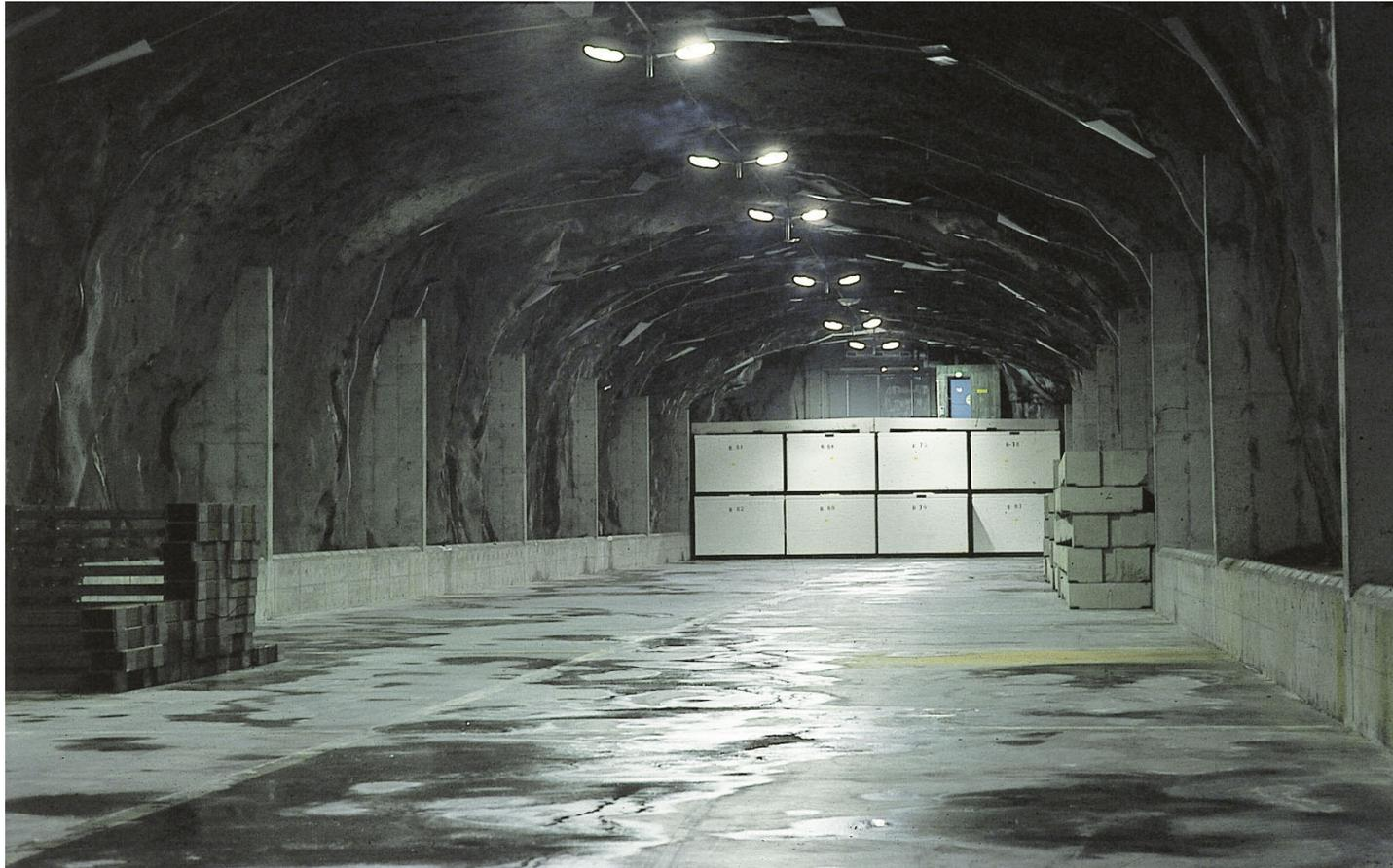
*Rock chamber for low- and intermediate level waste
