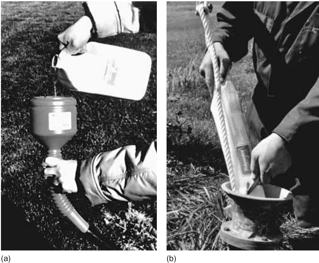
Figure 4-9 (a) Cable lubricant can be poured directly into the conduit before pulling. (b) For larger conduit, lubricant can be spread by pulling prepackaged bags through the conduit. Courtesy American Polywater Corporation
