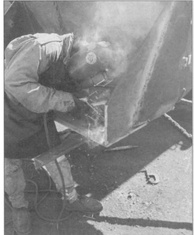
1.6 The construction and repair of heavy equipment and farm machinery would be nearly impossible without welding. Arc welding is usually used, as here modifying the front of a dirt scoop on a John Deere, where welding is outdoors and on heavy plates.
