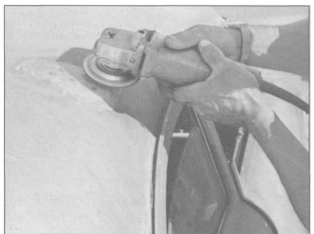
8.38 After the pulling, the stud heads are easily ground off without distorting the metal, and there are no holes left to fill in, as with conventional methods.
