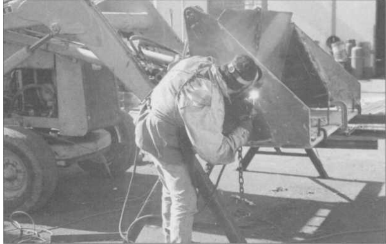
2.13 In farm and construction equipment repair, most work is done with oxy-acetylene cutting and arc, or stick, welding. Arc welding is not affected by wind outdoors, and is able to join or repair very thick materials.
