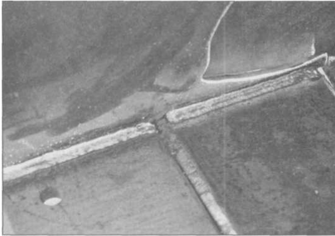
4.22 Here half-inch plate on the sides was welded with one pass, but a gap was left where the one-inch, beveled lower plates join. The bigger plate will be welded with several passes and strength is improved if the joint starts all the way at the ends.
