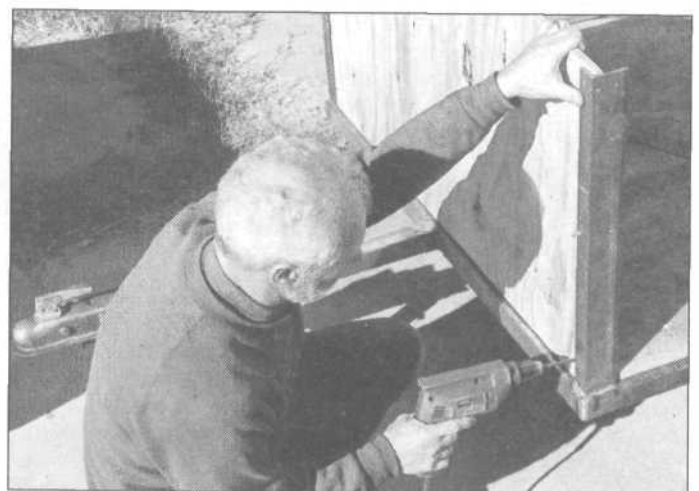
9.29 The front panel is attached with carriage bolts through the angle-iron posts. The posts were pre-drilled before welding on, because they are much easier to drill in a drill-press than once they are welded in place.
