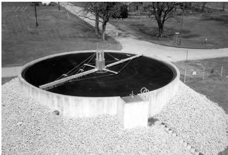
Figure 16.5 Attached-growth wastewater treatment system.
