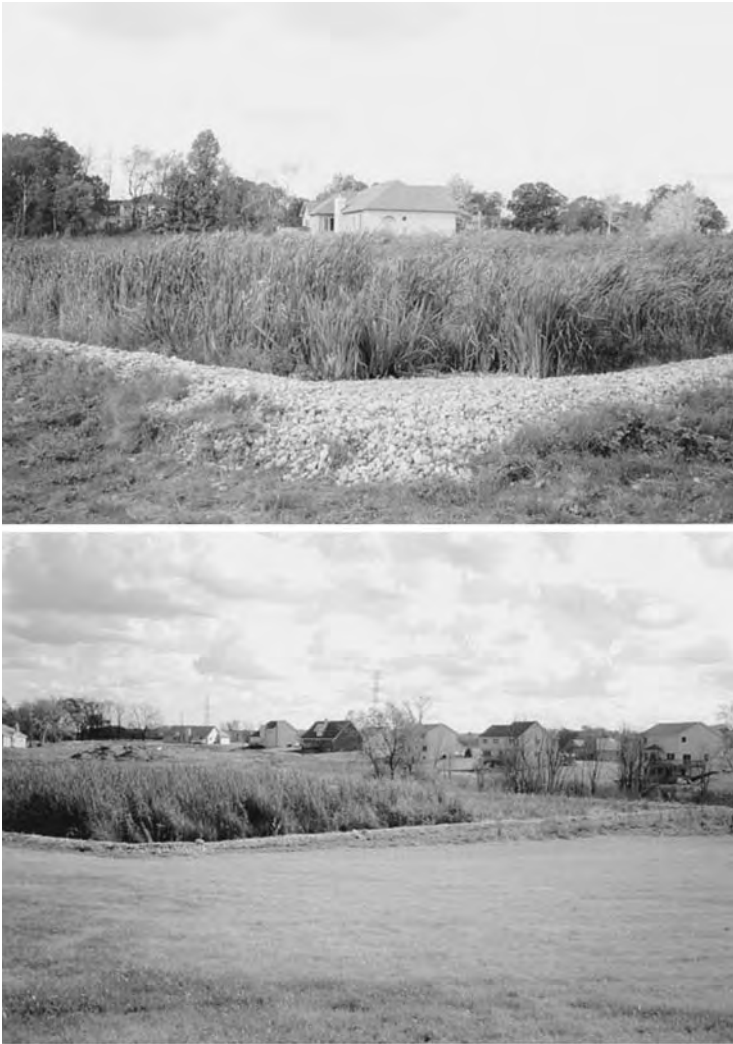
Figure 16.35 Constructed wetland wastewater treatment systems.
