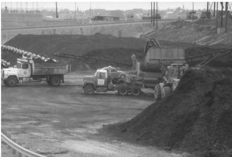
Figure 16.51 Sludge composting: (a) aerated piles; (b) bulking agent screening and recovery.
