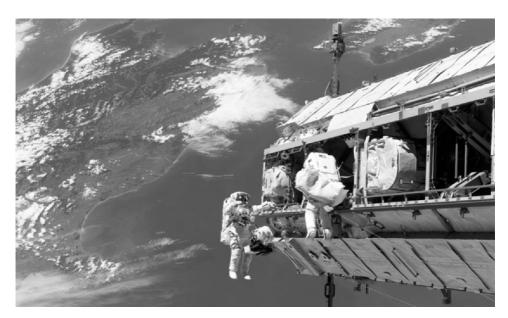
Figure 9.1 High above New Zealand, astronauts Robert Curbeam and Christer Fuglesang work to attach a new truss segment to the ISS on December 12th, 2006. Courtesy NASA.
