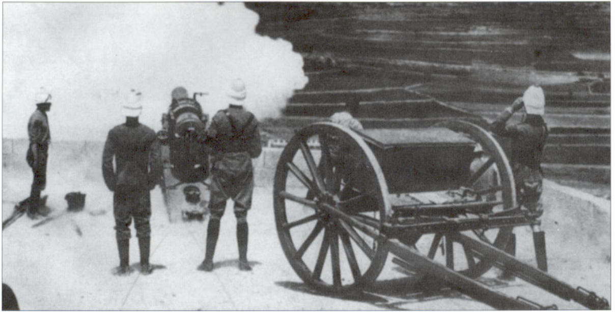
Maxim machine guns on the Victoria Lines. The field carriage mounting conferred mobility and allowed ammunition to be carried in 16 boxes, each containing 250 rounds. Because of their high profile, field carriages were of dubious use when the enemy was equipped with artillery and magazine rifles. They therefore tended to be deployed in colonial warfare scenarios against 'savage' (i.e. poorly armed) enemies. (Photo courtesy of Richard Ellis Ltd.)
