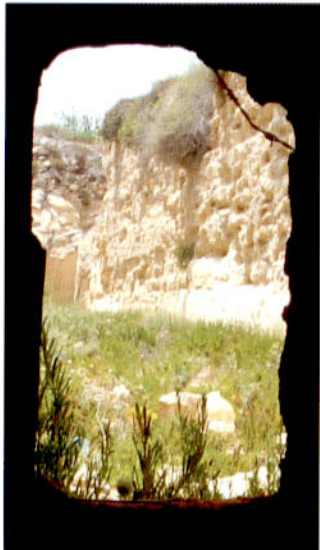
ABOVE LEFT Sunk into a drop-ditch (a ditch within the main ditch but at 90 degrees to it) this view through a caponier loophole shows the virtual impossibility of attackers being able to survive in, or get across, the main ditch. Because of the drop-ditch, the exposed portion of the caponier presented only a small target. (Courtesy of P. Evans)
