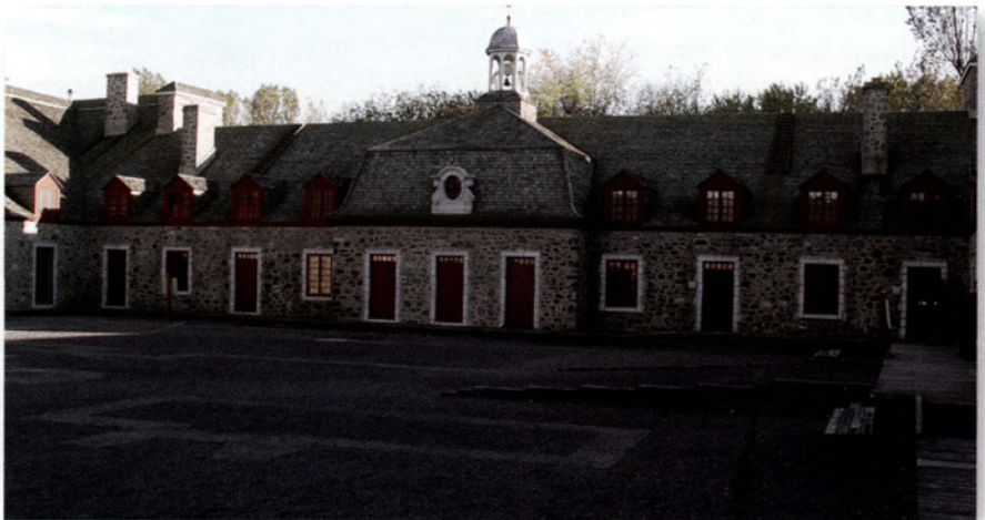
Interior of Fort Chambly. The chapel roof is restored according to its appearance as rebuilt in 1750. The marks on the ground of the center courtyard indicate features of the 1702 fort found during archeological work. At lower right, a line of logs from the stockade and buildings at the center.
