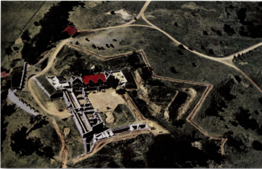
An early bird's-eye view of Fort Carillon at Ticonderoga, NY, taken in the 1920s. This colored photograph shows the fort before most its reconstruction, notably the stabilized foundations of buildings on the south and east sides. The slanting side walls of the buildings are clearly visible. Private collection.
