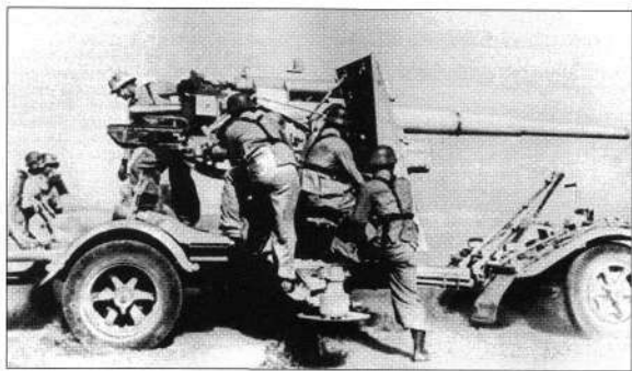
A heavy Flak 18 88mm getting ready to fire against a ground target while still in its towing arrangement. It equipped the Lufwaffe's schwere Flak Batterien (heavy anti-aircraft batteries) that, along with the leichte Flak Batterien armed with the 20mm Flak 38, formed a Flak Abteilung . Each Abteilung had three schwere Batterien for a total of 18 Flak 18 pieces. (Carlo Pecchi Collection)
