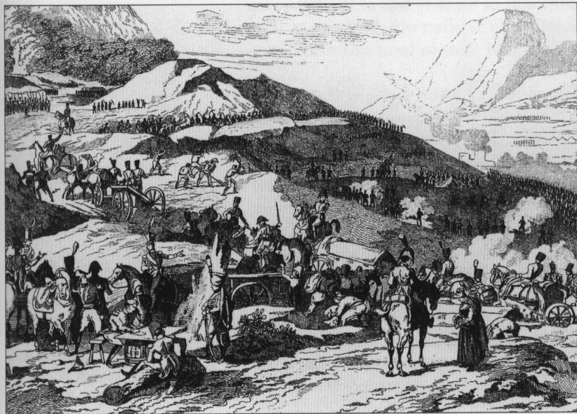
Field artillery setting up before a battle, c. 1805. Note the many men handling picks and shovels building the field fortifications for the batteries. (Print after Martinet)
