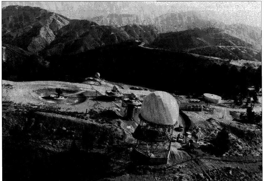
Nike-Hercules integrated fire control area at Nike site LA-04 at Mt. Gleason in the Los Angeles defense area. The radars in a row are (from the bottom) the High Power Acquisition Radar (HIPAR) atop the pedestal tower and protected by a radome, the Target-Ranging Radar (TRR), the Target-Tracking Radar (TTR), and the Missile-Tracking Radar (MTR). Standing alone at the left side of the photo is the Low-Power Acquisition Radar (LOPAR). (Courtesy Col. Milton B. Halsey, Jr.)
