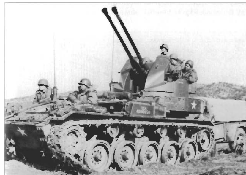
An M19 40mm MGMC moves to the front in Korea, towing a standard M28 1-ton ammunition trailer. In Korea, the M19 was mainly used to provide fire support against ground targets owing to the absence of enemy aircraft after the summer of 1950. (US Army)
