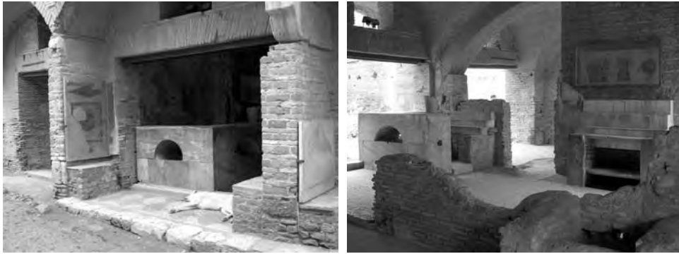
Figure 19.1a and b Ostia, tavern on the Via di Diana, exterior view. Note street-front bar and benches out front. The open nature of the place suggests the vibrancy of street life in Roman towns (b) Ostia, tavern on the Via di Diana, interior view. Note the painting on the wall advertising food available for sale. The shelving below probably displayed fresh items, as in modern Italian restaurants
