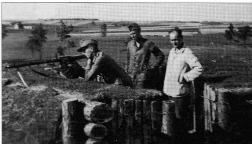
A raised machine-gun position. As winter approached the Germans raised trenches so that the fire position for the weapon would be just above the height of the snow when it had fallen. Note the timber reinforcement of the position prepared well in advance.
