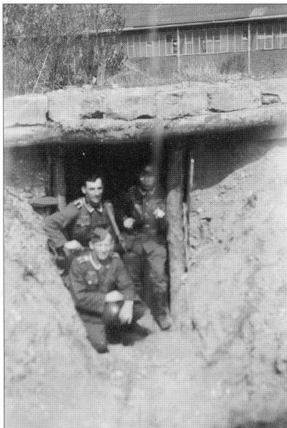
Another section position, well dug in with overhead cover, this time of thick concrete blocks.
