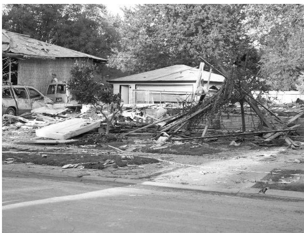
All that remains of a house after the gas line ruptured during a flood. The explosion also destroyed three adjoining houses.
