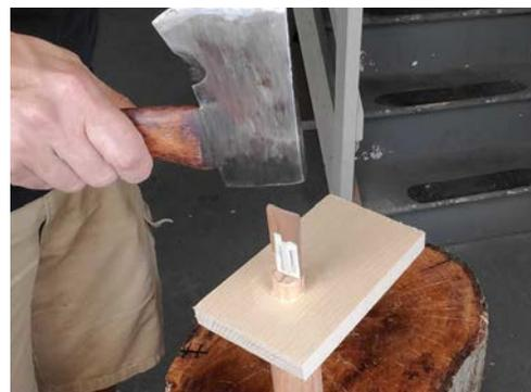
*I put glue around my tenon before inserting it in the mortise. Now, I've got glue on my wedge and I'm inserting it into the slit and tapping it home with the back of my hatchet.*
