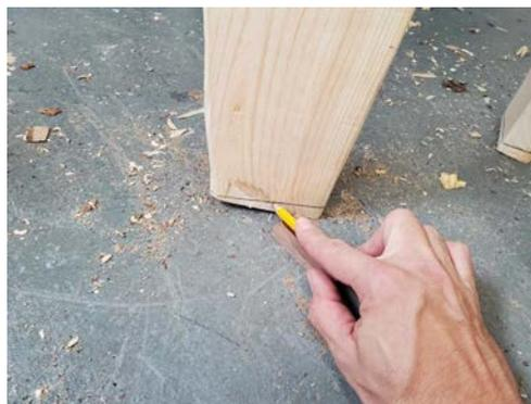
*A pencil and a scrap of wood will make a marking tool that scribes the plane of the floor onto your legs. Crosscut this line and your leg will sit steady on the floor.*
