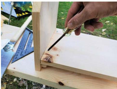
*Screwing through the bottom and into the cleats will tighten up the structure. In the picture, you can see a small gap between the bottom and the end. As I tighten my screw, that gap will close.*
