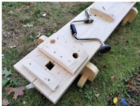
*Before I glue in the legs, I'm screwing on the small battens. These are made from the extra legs I didn't use. I put one batten in the middle of the bench and one at either end. The exact locations don't matter.*
