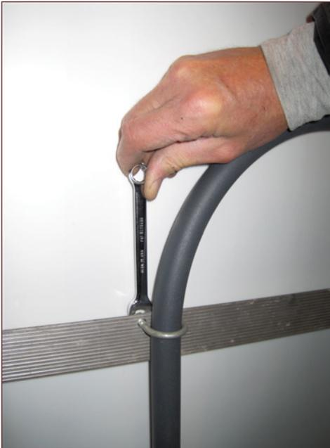
***Tightening nut on U-bolt securing panel to hand truck frame. Background is white plastic rear of photovoltaic panel.***
