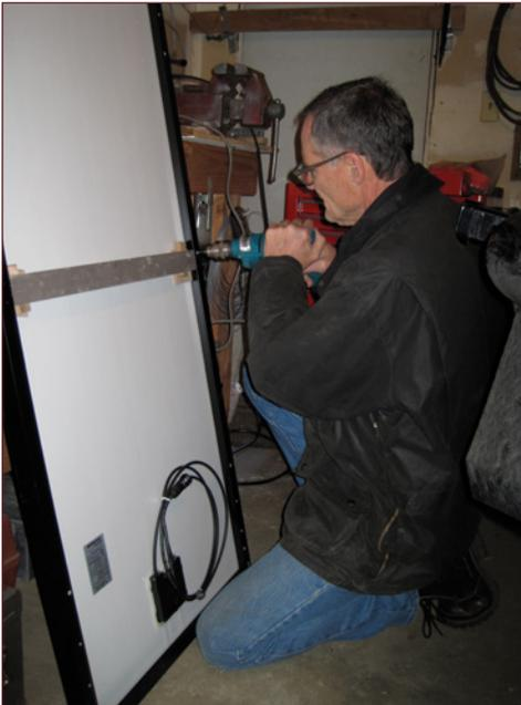
*Drilling holes through photovoltaic-panel frame and horizontal aluminum support. Wood wedges hold aluminum support in place during drilling.*
