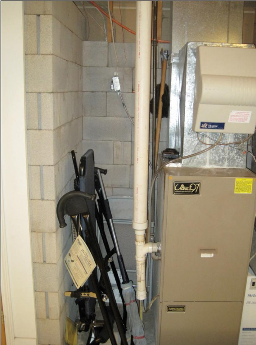
***When completed, author's safe room looks like it was built as part of the house. Using half-blocks enables staggering the full-size concrete blocks.***
