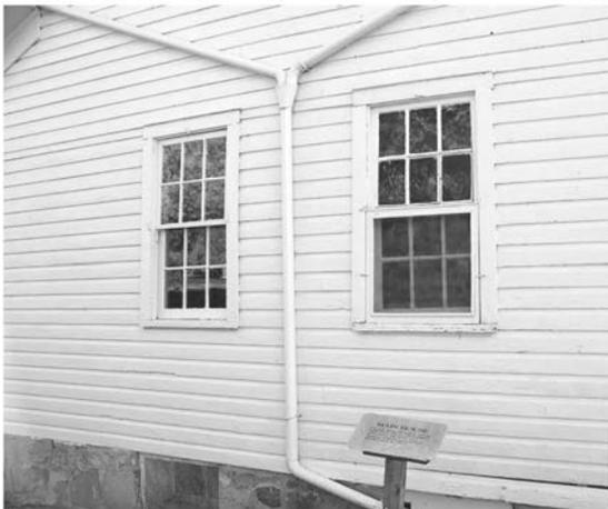
Amish home with gutters routed to basement cistern. A pump in the kitchen brings the water to the sink.
