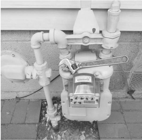
Keep a wrench close to your gas meter. *Caution:* After you turn the gas off, you should have the gas company turn it back on.
