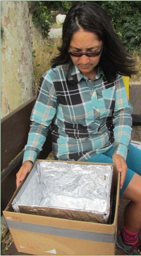
*Insert the smaller box into the larger box. Pack the space between the boxes with crushed newspaper. Make sure to insulate the space at the bottom.*
