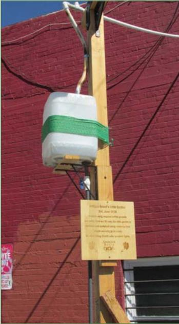
*Water that flows out of the AC unit at Antigua coffee shop flows into this bucket, where it then flows by gravity into the garden.*
