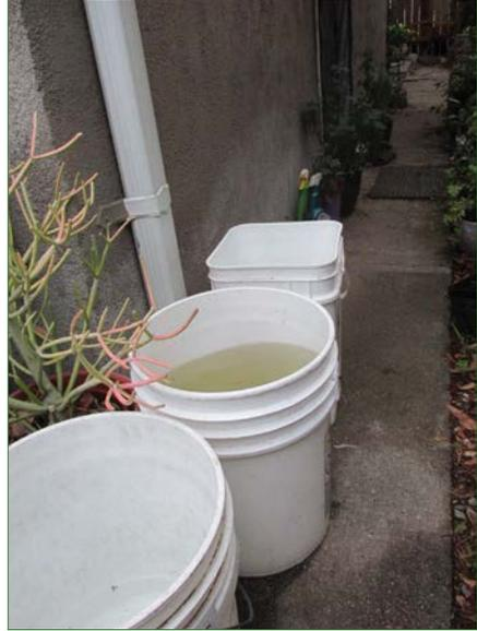
***These buckets were placed close to the house, directly under a rain gutter which drains into the buckets. The rainwater is then filtered before using.***
