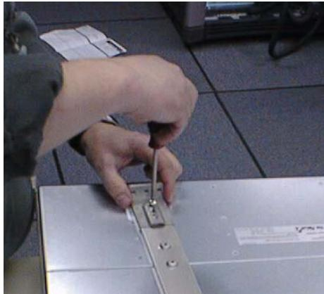
**Figure 2-3** Attaching the Inner Bracket
