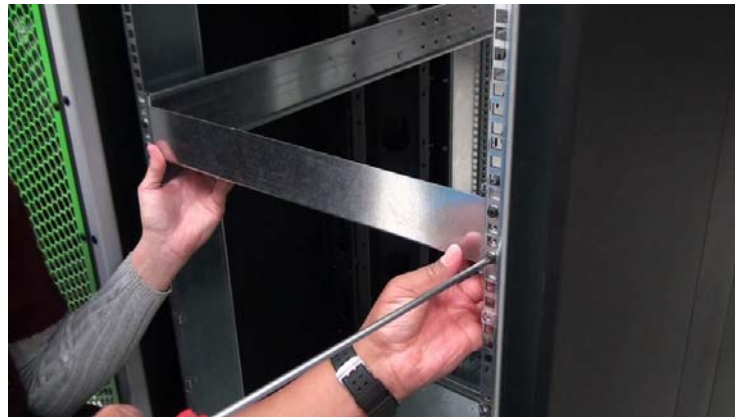
Figure 1-16 Adjustment Using the Alignment Tool
