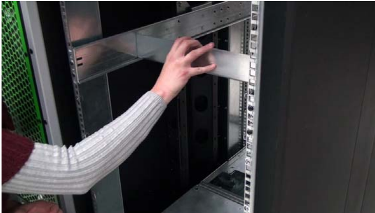
Figure 1-17 Slide the Alignment Tool from Front to Back
