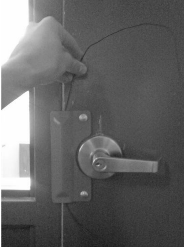
Figure 9-15 Bypassing shim guard with thin cable
