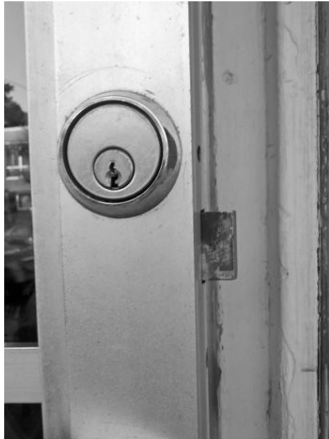
Figure 9-4 Deadbolt-type straight plunger
