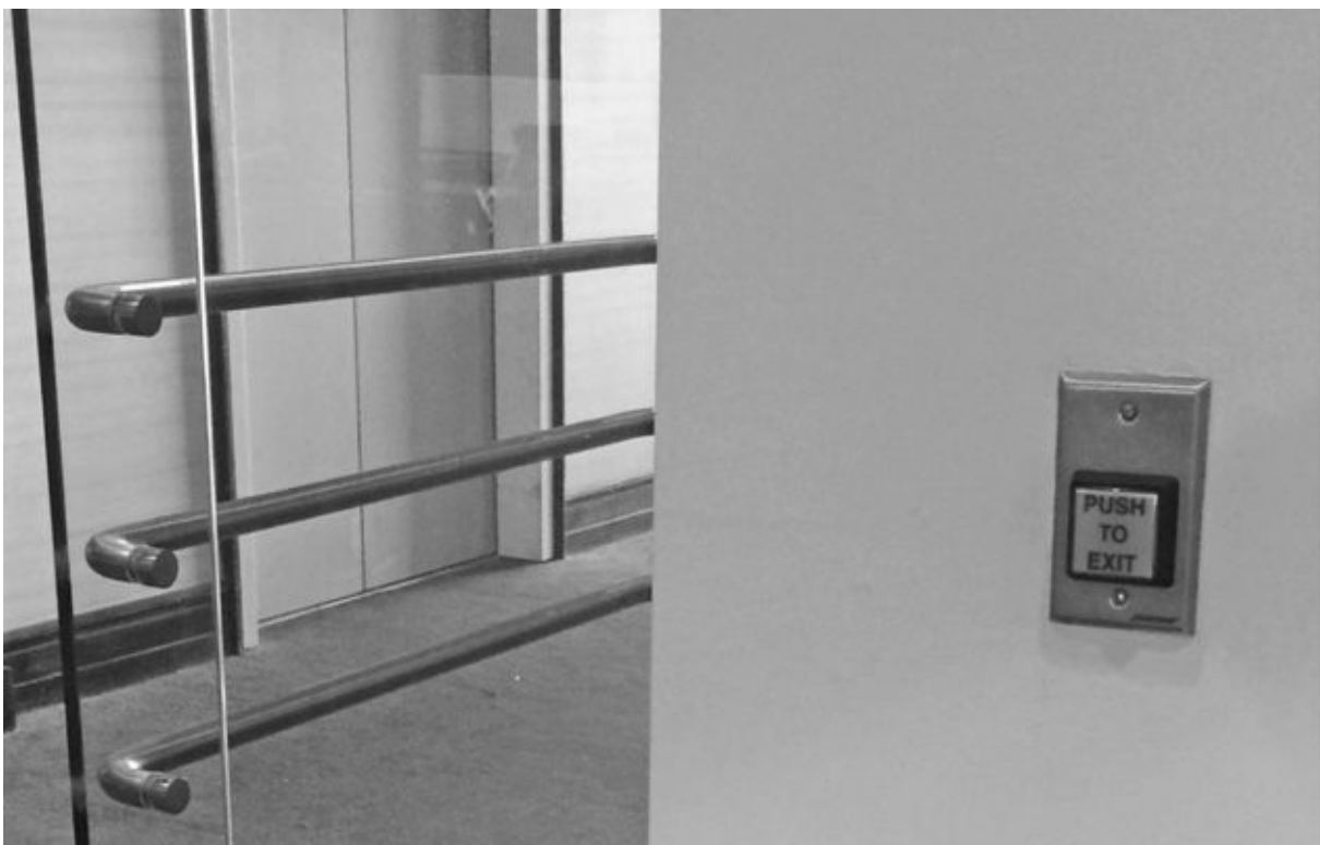
Figure 9-16 Push-button door exit
