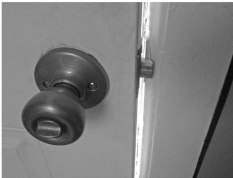
Figure 9-3 Door plunger mechanism and door strike plate
