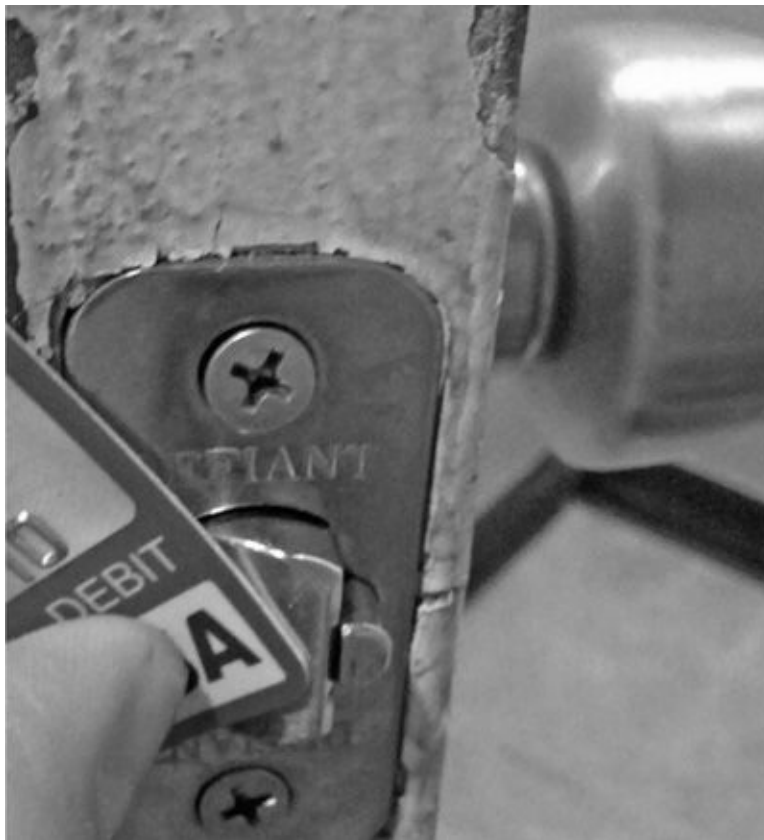
Figure 9-13 Shimming lock plunger with credit card
