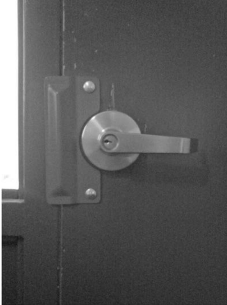
Figure 9-14 Shim guard blocking access to plunger
