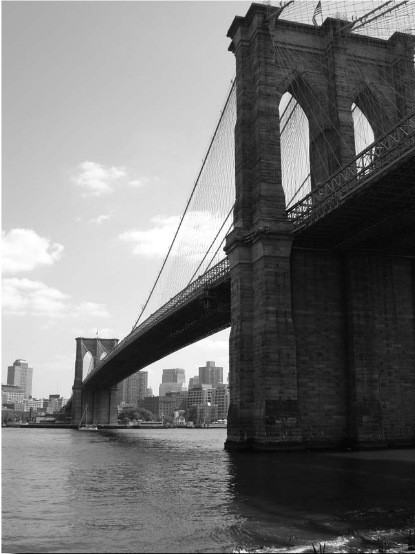
FIGURE 1-1: The Brooklyn Bridge from its base.
