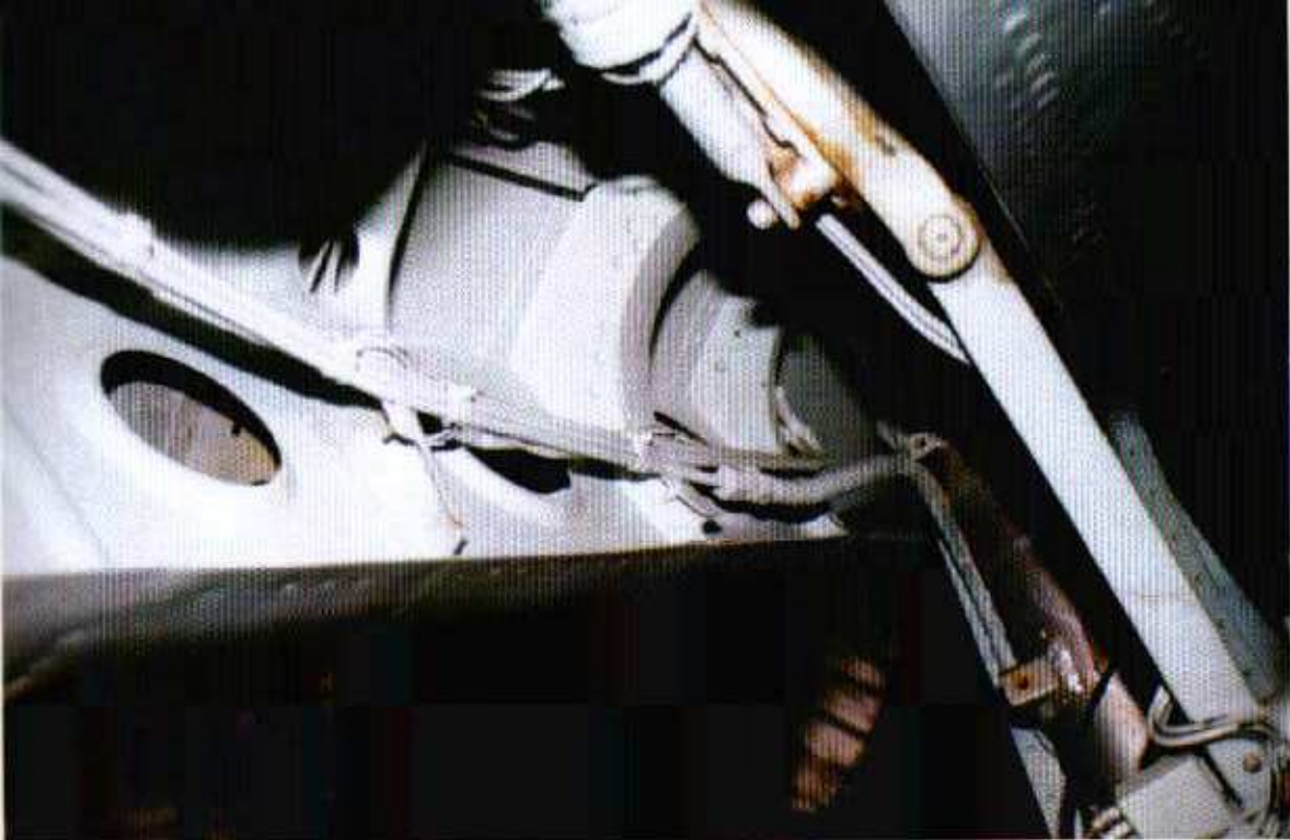
(Above) The construction of the starboard wheel well's forward wall with its electrical and brake lines are seen to advantage. (Author: Ryle)
