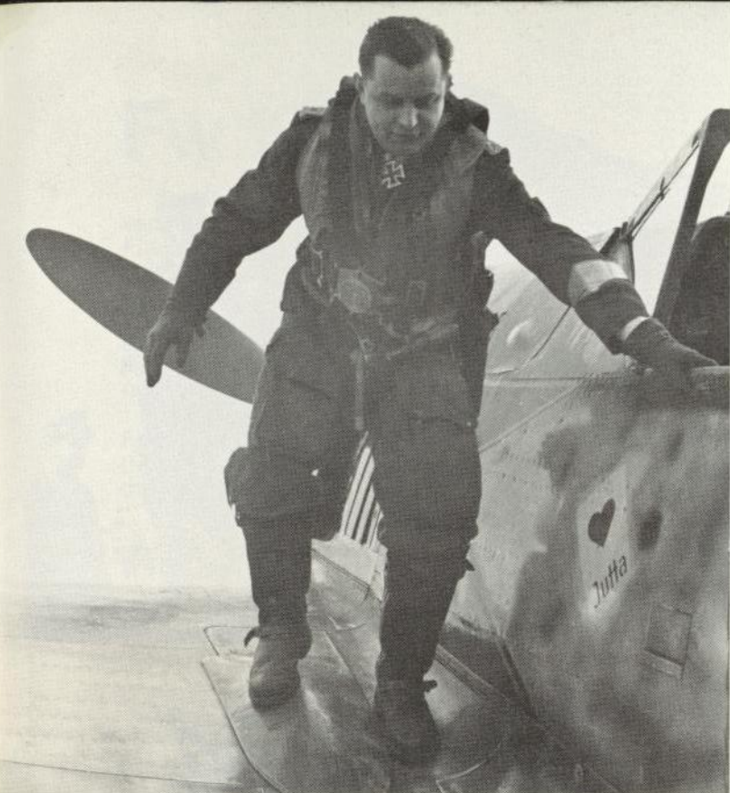
Priller wears a plastic map holder on his left forearm. The bulged panel he is standing on houses the MG 151 wing root cannon that was first introduced on the Fw 190A-2.
