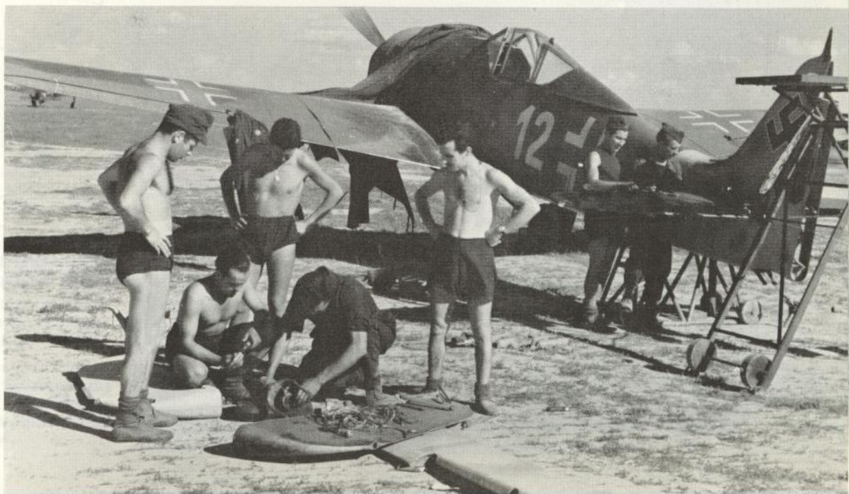
Priller wears a plastic map holder on his left forearm. The bulged panel he is standing on houses the MG 151 wing root cannon that was first introduced on the Fw 190A-2.
