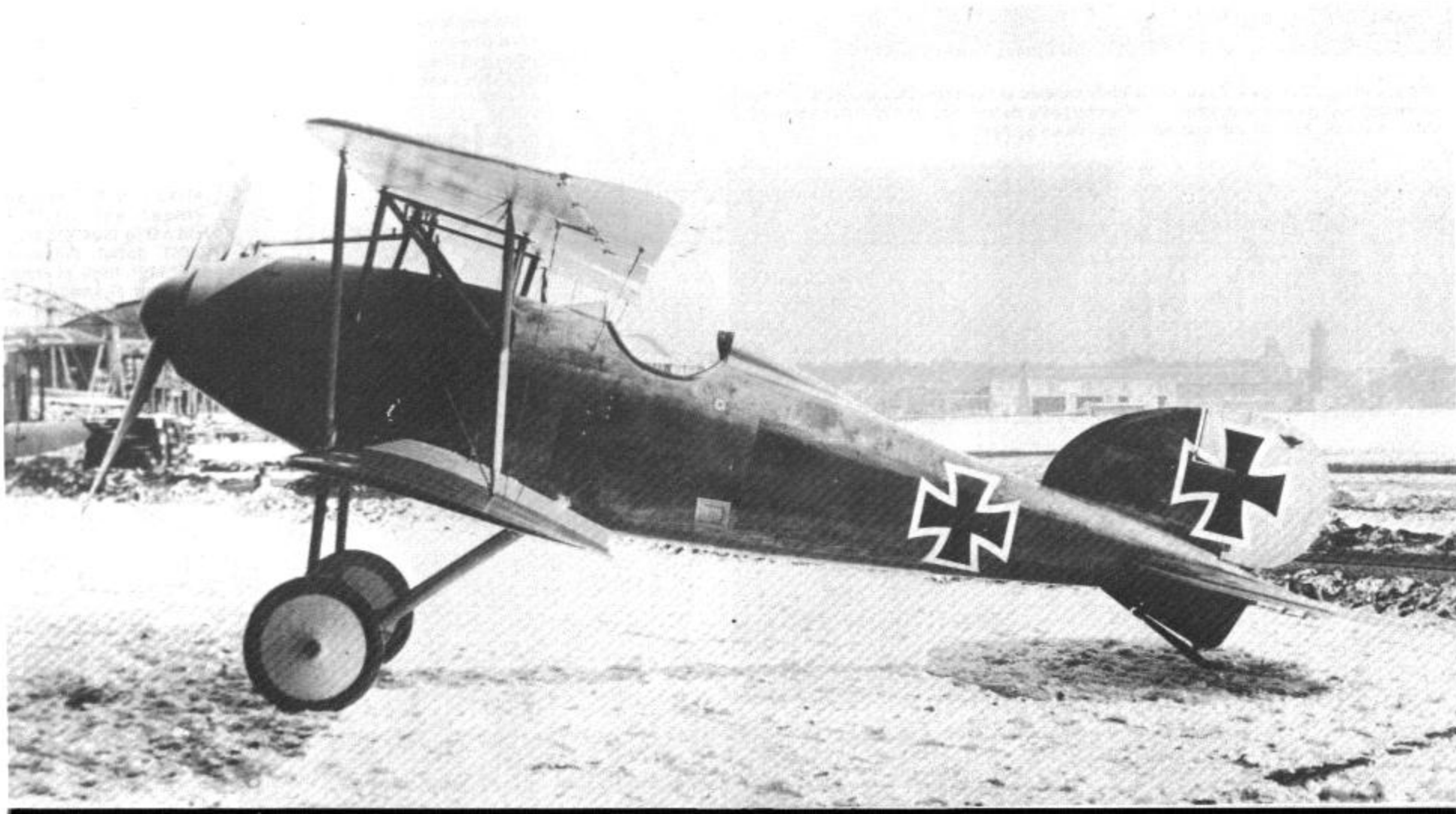
The only verified Albatros D.IV prototype. Note small headrest, square balance on rudder, larger chord of lower wing, parallel interplane struts and completely cowled engine. Of three examples ordered, this is probably the only one completed.
