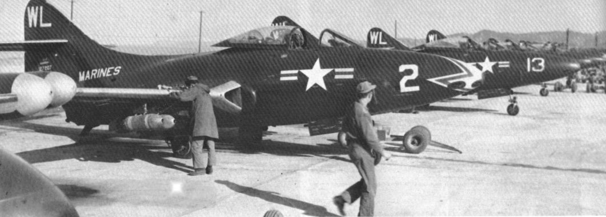
F9F-2 (127207) of VMF-311 at K-3 (Pohang) base, Korea. No. 2 has Red and White trimmed nose...Panthers are being armed with bombs and 20mm. Fall 1952. (USMC)
