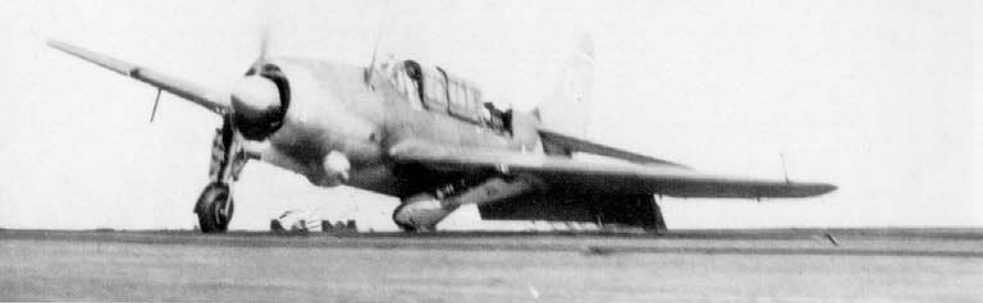
Another endearing quality of early Helldivers was frequent main gear collapse. Here, '13' plants its left wing on landing, Essex, 20 May 1944. (USN/NARS)
